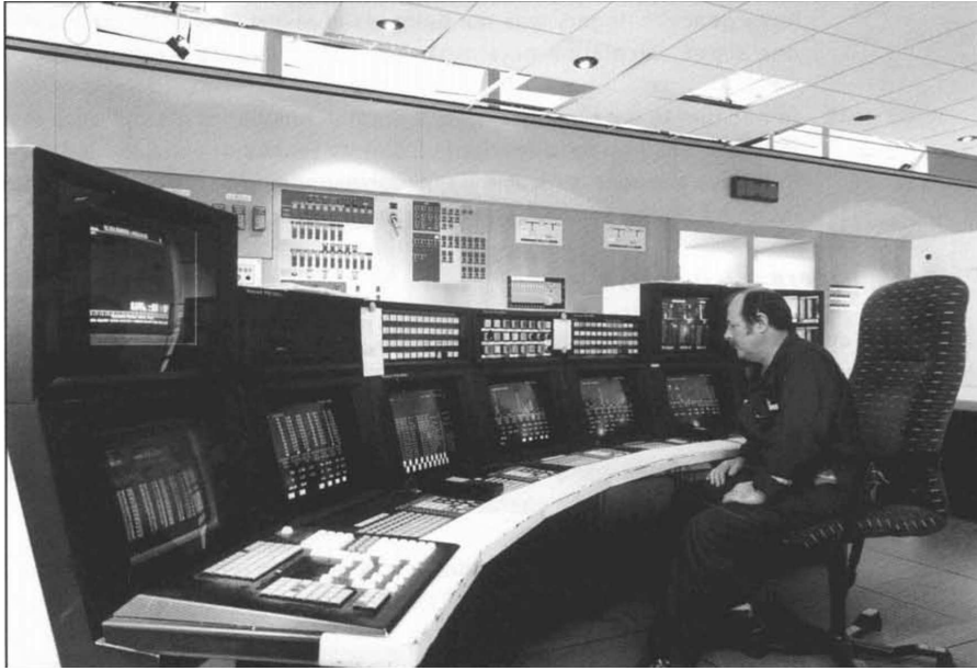
Figure 2: One workstation in the main control room of the Texaco refinery. Image produced from [77]
